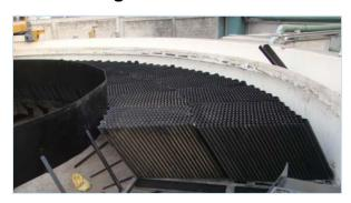
For higher sludge loads and smaller inner diameters we recommend installing the TUBEdek® modules radially. This can be done by cutting the modules into segments like pieces of a cake. The form of the edge profiles allows for an installation without dead ends.
