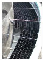
TUBEdek® lamella clarifiers can be installed tangentially in a ring at the outer rim of the tank. For this configuration, the width of the ring may not exceed 3 m and the inner diameter of the tank has to be larger than 12 m.
