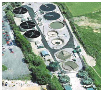
Municipal WWTP Ernesettle, Great Britain
